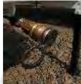
12 Volt Exterior Lighting at Patio w/ Interior Switch
