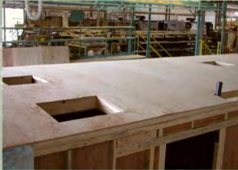
Tongue & Groove Plywood Floor Decking & Plywood Roof Deck
